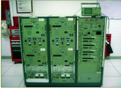
**Figure 4.** AN/FPN-54 Timing Rack where the LORAN pulses are generated for amplification in the AN/FPN-45 vacuum tube transmitter. Photo courtesy of ETC K. Anderson.
