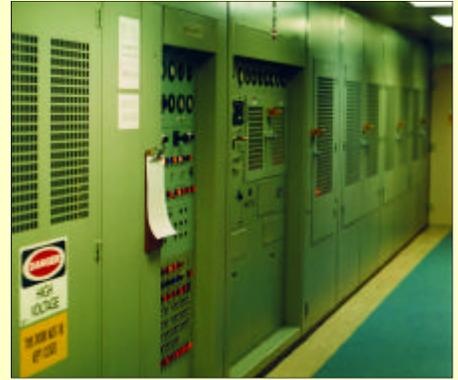
**Figure 6.** One of the two AN/FPN-45 transmitters on air, cranking out 1.6 megawatts.
