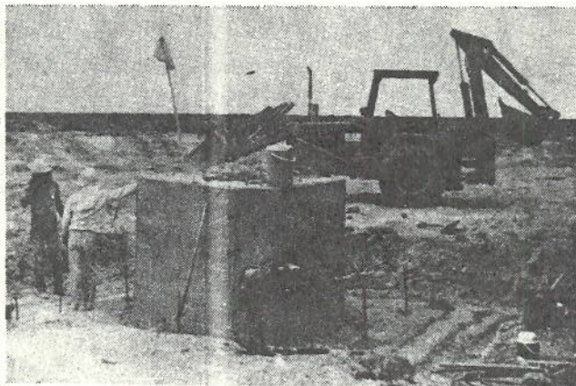
On going construction at the LORAN job site.
