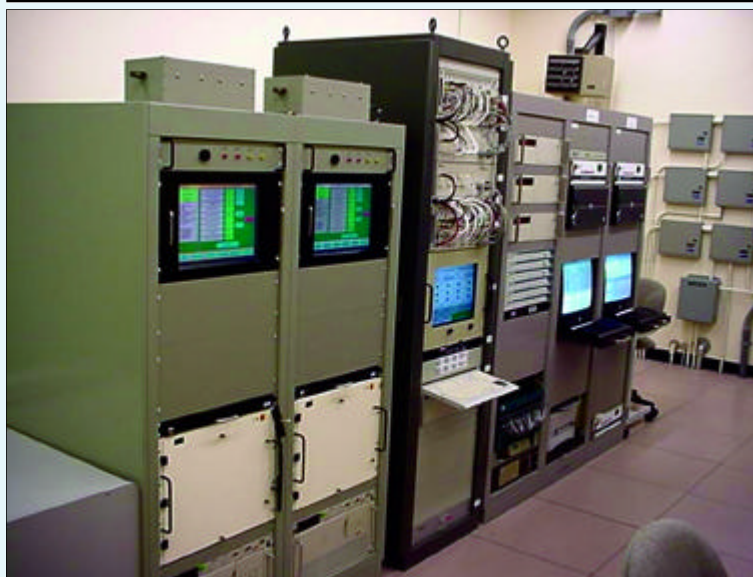
Figure 1. The frequency/control equipment for the solid-state transmitter. The two left racks are the TCS, then there is the TFE, the AUX rack with three cesium beam frequency standards, and two RAIL racks on the right. Love that alphabet soup! Photo courtesy ETC K. Anderson.
