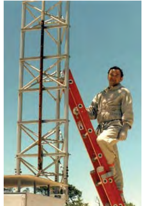
Pete Hennings ('62) mounting an energized Loran-A tower, wearing a conductive suit
