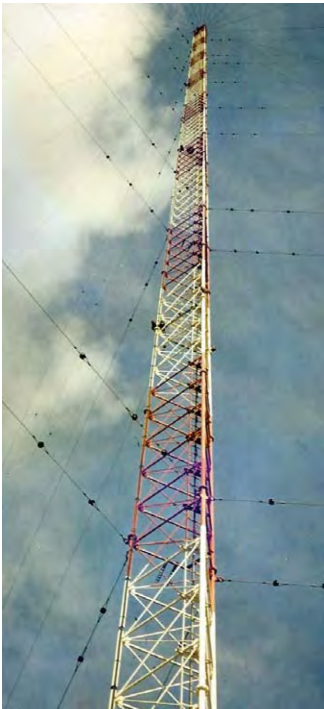
Typical 625-ft. Loran-C tower (Kargabaran, Turkey)
