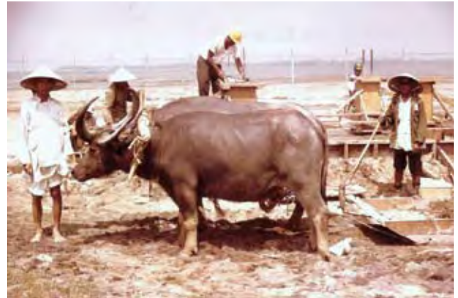
Specialized construction equipment, LORSTA Tan My (Vietnam)
