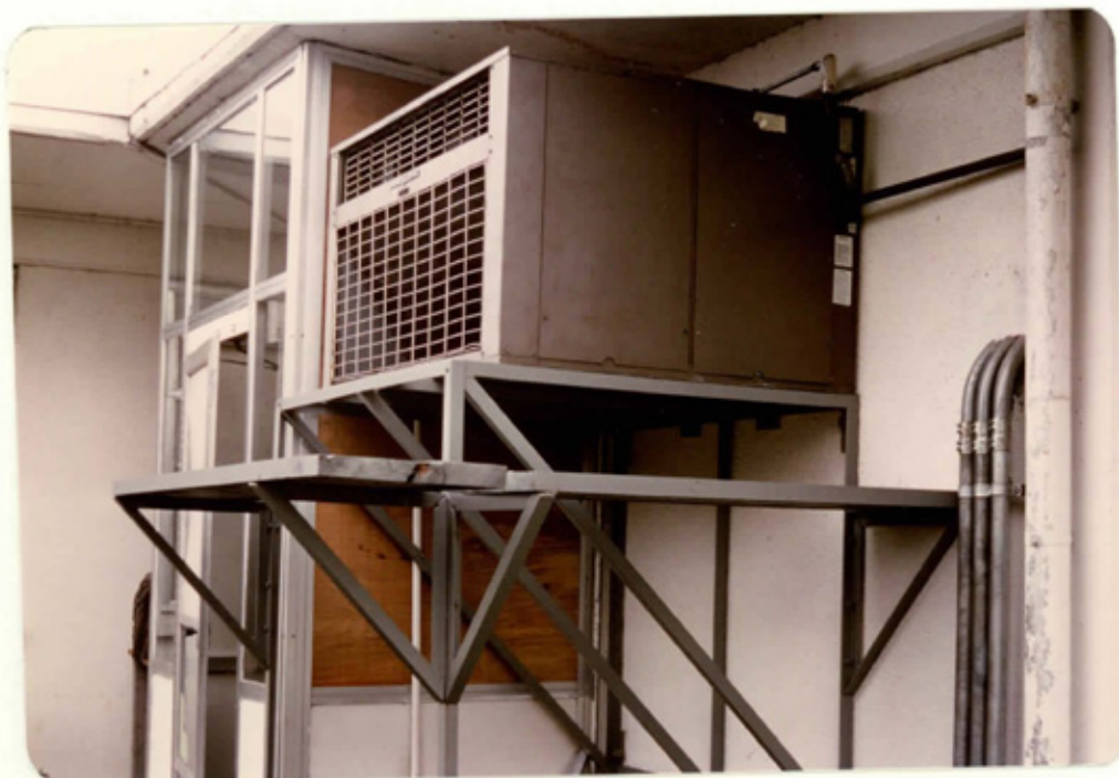
4. Station has built walkways around heat pumps/units
