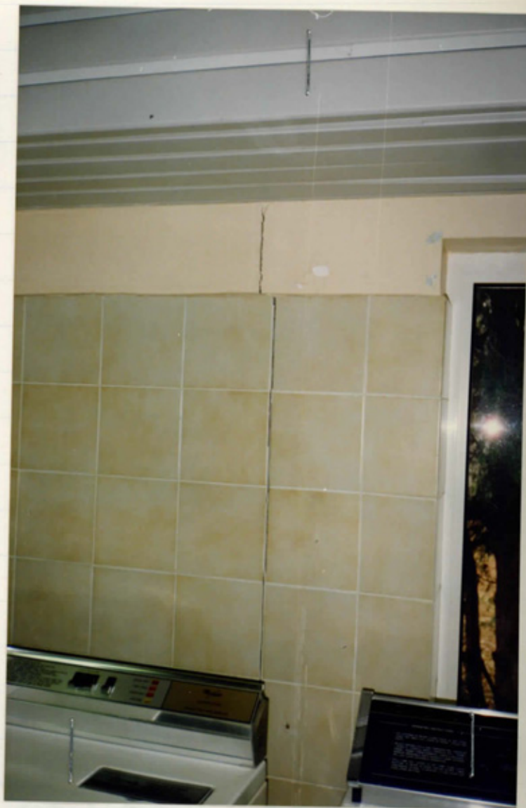
Photo #5 Laundry Room Interior Side Wall Crack
