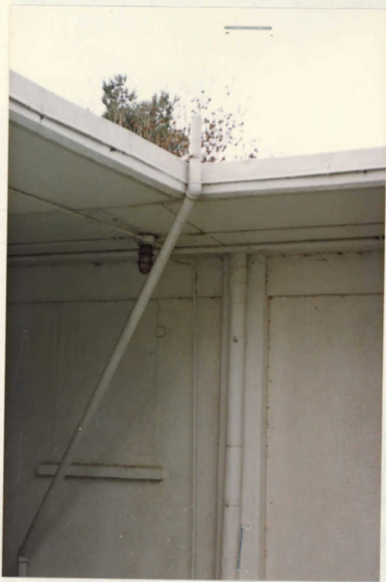
Photo #1 Sewage Vent Pipe - Barracks Bldg.
