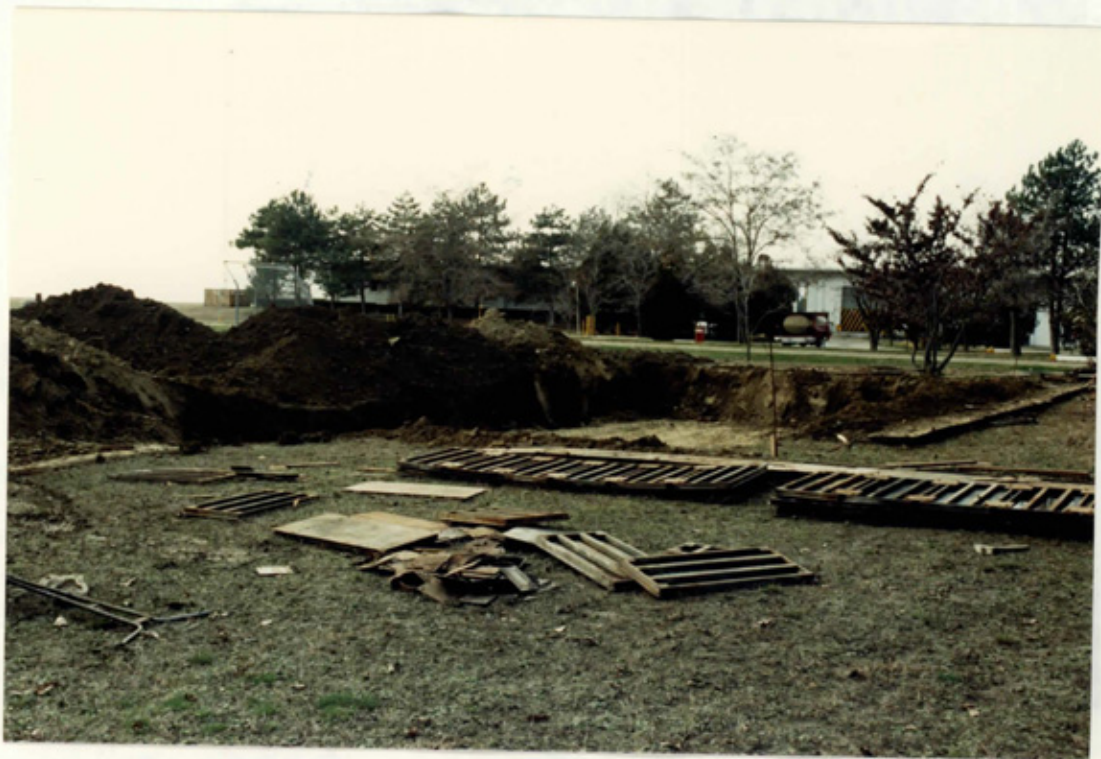
REHAB: New COQ. Excavation for COQ foundation.
