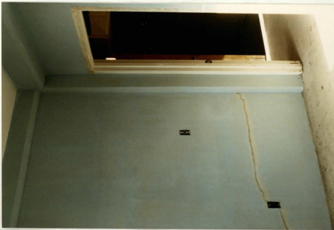
REHAB: Barracks rooms (Petty Officer Wing). Sealing of cracks and painting
