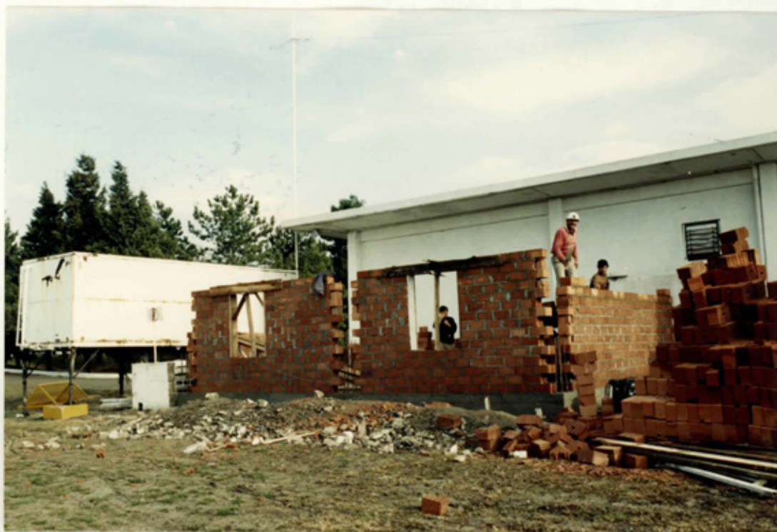
REHAB: Construction of inspector's office. This building will be used as office space during the rehab, and then turned over to the Coast Guard as a new storage facility.
