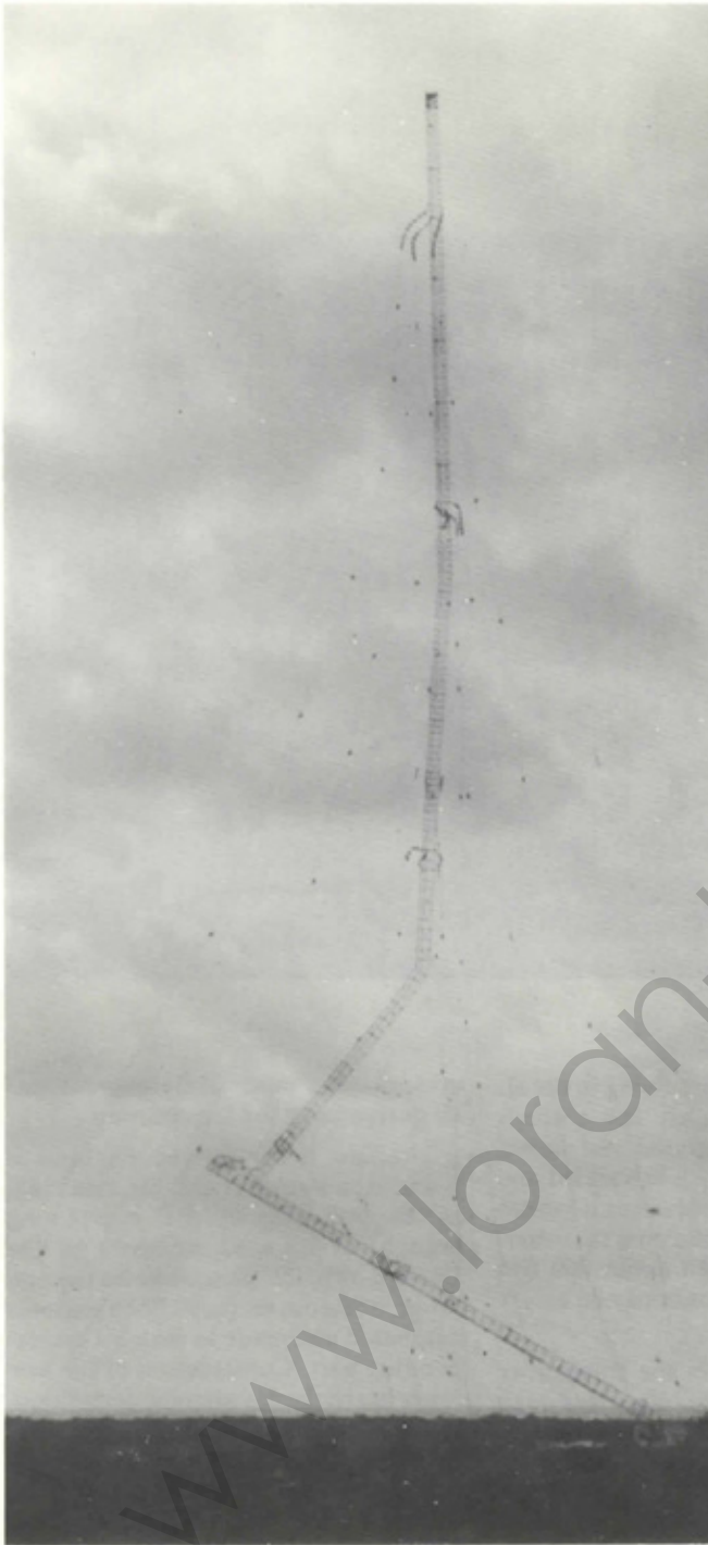
The 1,350-foot-high tower begins its downward descent.
