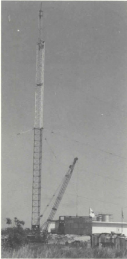
The new tower goes up.
