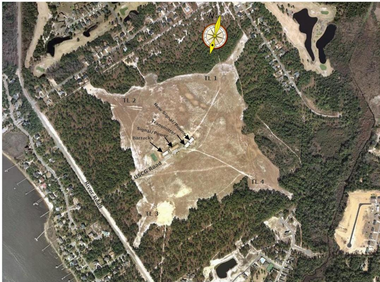
Figure 16. Map of USCG Carolina Beach LORAN-C station with buildings and towers. Source: Bing Maps.
