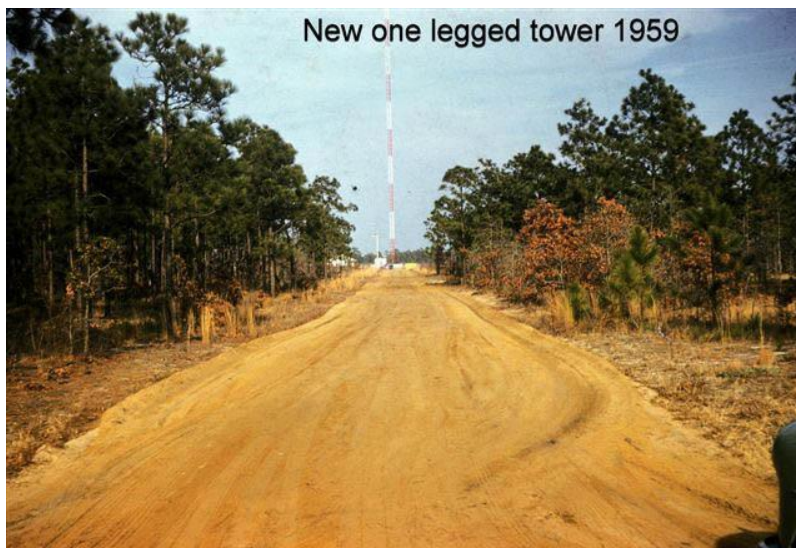
Figure 21. Photo showing the single guyed tower (c. 1959). (Available online at: http://www.loran-history.info/carolina_beach/carolina_beach.htm ).
