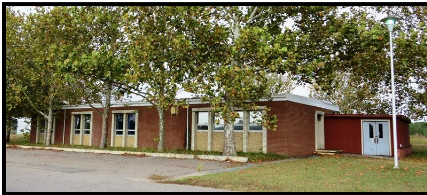
Figure 10. The Barracks building (c. 1971)
