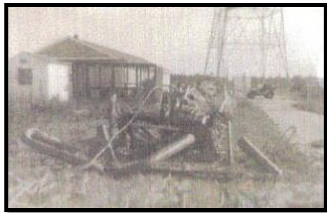
Figures 18 and 19. Hurricane Helene photographs. Picture on the left shows upper section of the tower has been broken; Picture on the right depicts the top third of the tower on the ground. Source: USCG website available at: http://www.loran-history.info/carolina_beach/carolina_beach.htm
