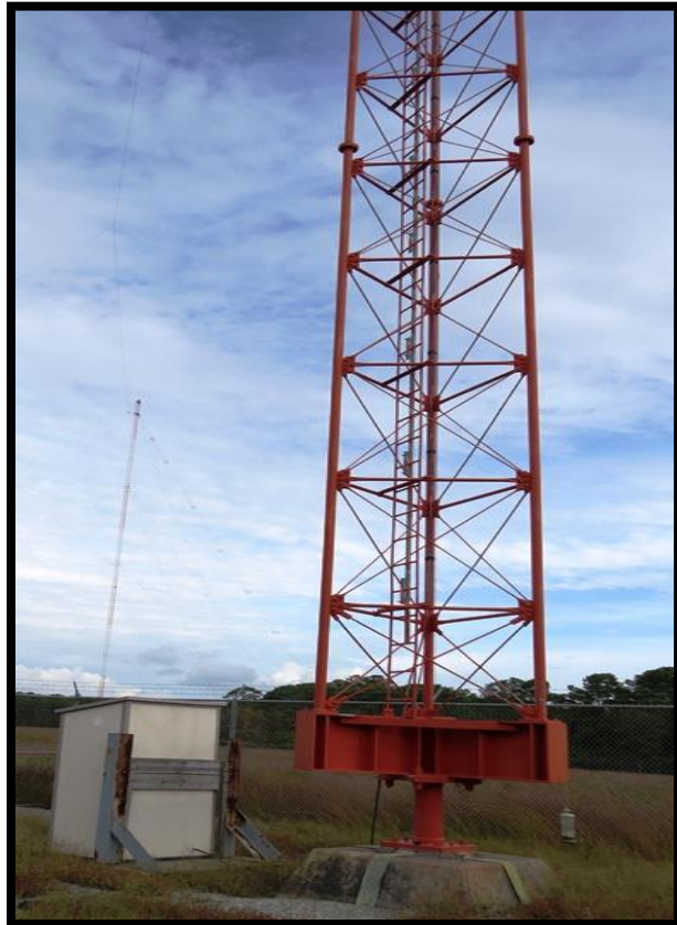
Figure 3 and 4. Top of LORAN-C tower (TL1), and tower base (TL4), USCG Carolina Beach LORAN-C station, Wilmington, NC.
