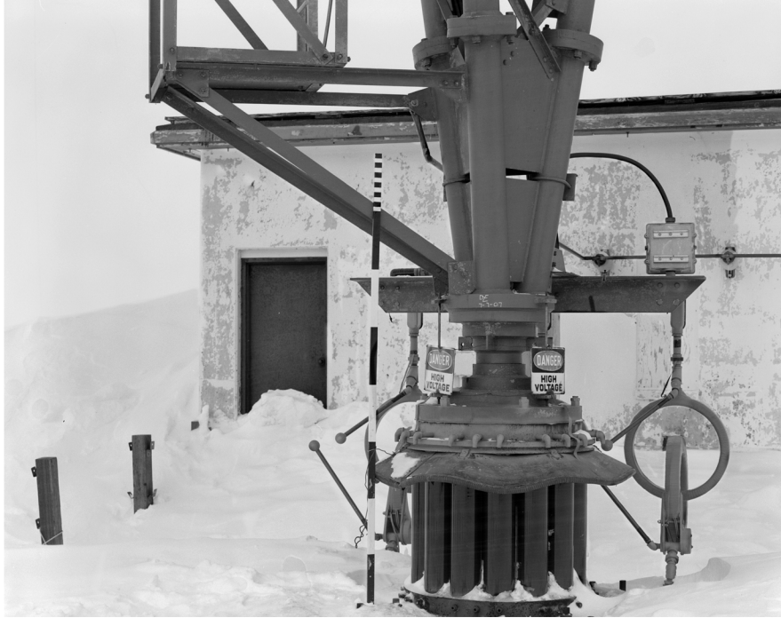
7. Tower base looking northeast
