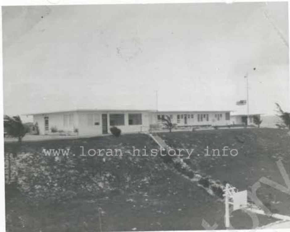
MAIN BARRACKS FROM BELOW
