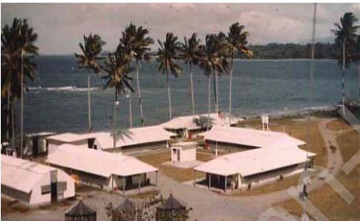
1956 Station rebuilt – Concrete Block Building construction (photo courtesy of Don Anderson / www.loran-history.info ) In the article listed below, Don tells about security duty and carrying arms when hiking. The article can be found @ www.loran-history.info/tarumpitao
