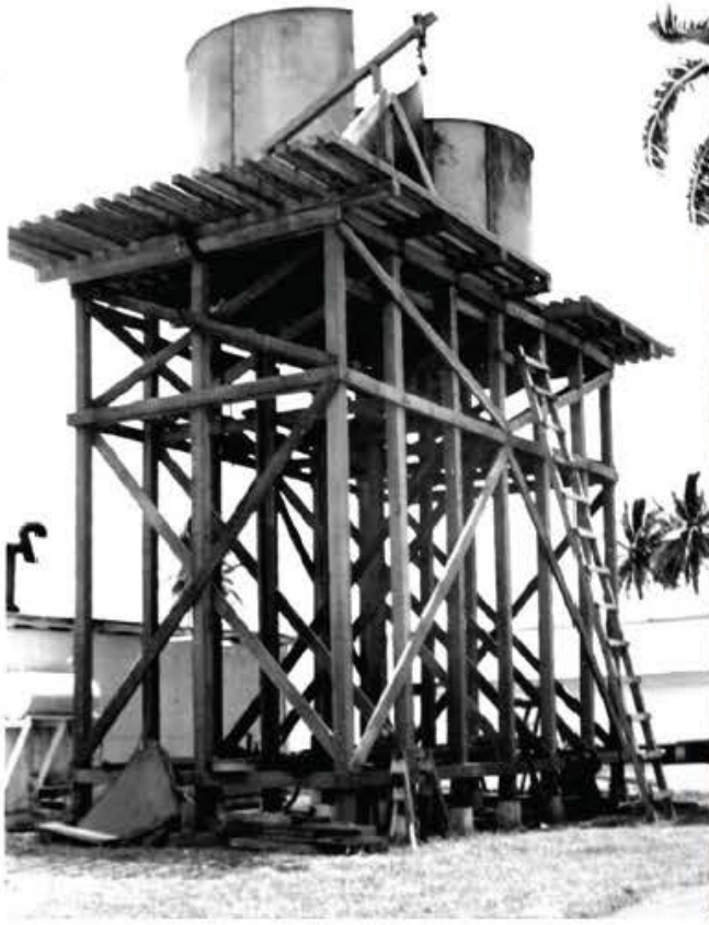
Rebuilding the water tower
